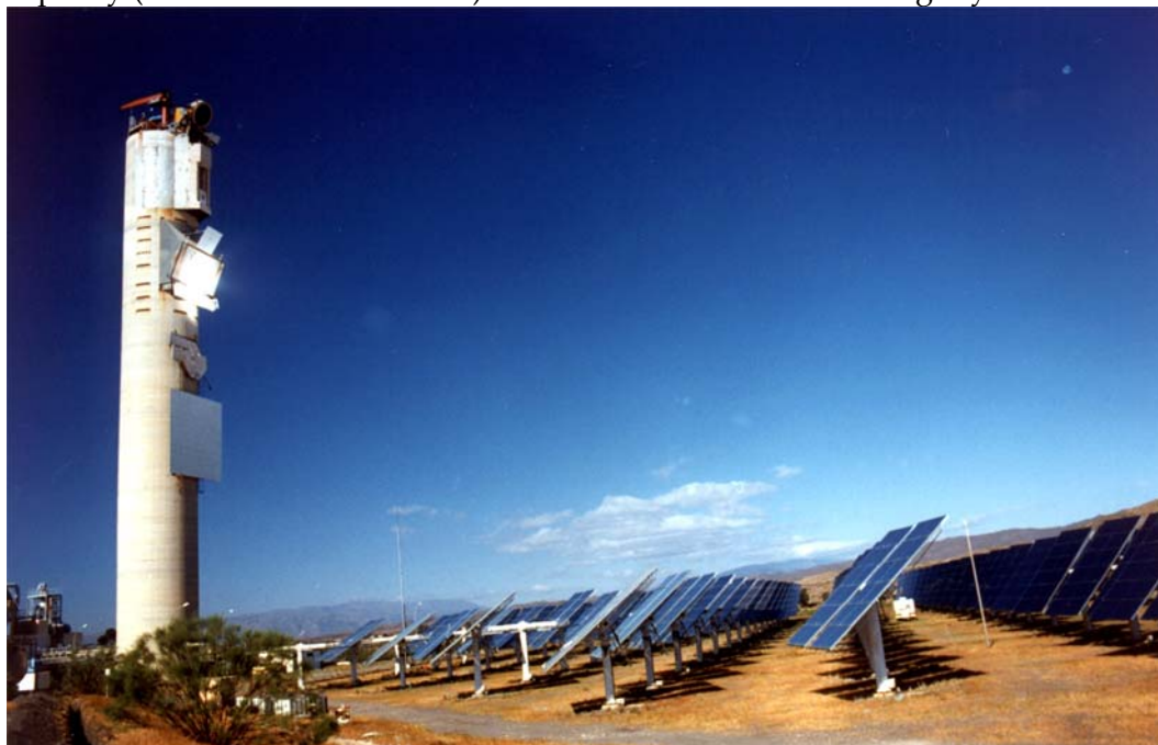
Figure 3. Detail of CIEMAT's 7-MWth CESA-I tower system and its 12000-m 2 heliostat field, located in Almería (Southern Spain).
